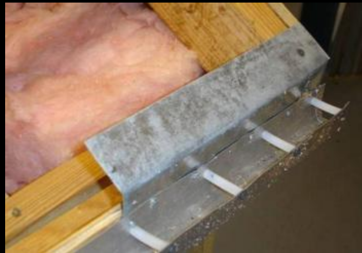
Flashing with galvanized or aluminum flashing
